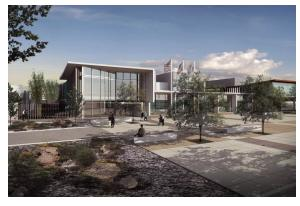
Building's design will support the concept of transparency to the community. As a practical solution for minimizing storm water run-off from the site, bioswales are located throughout the project. Bioswales will provide additional landscape areas to view from the offices and bring natural light into the building's interior spaces. The project is targeting LEED Silver certification.
