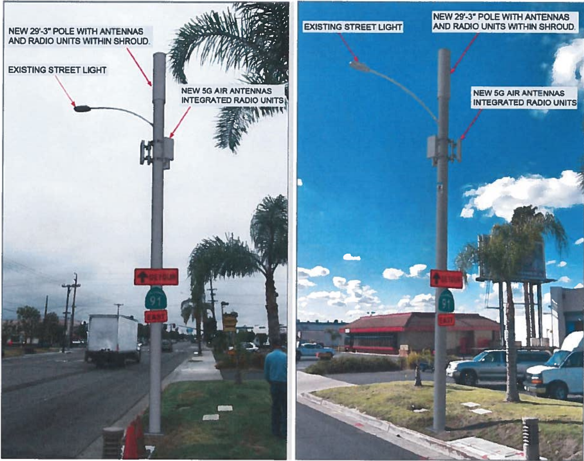
Pole shrouds, streetlight, radio units finishes to be as depicted in simulations.
