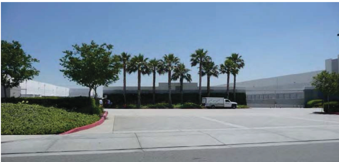
Figure 5-25 Example of Appropriate Ground Mounted Equipment Screening
