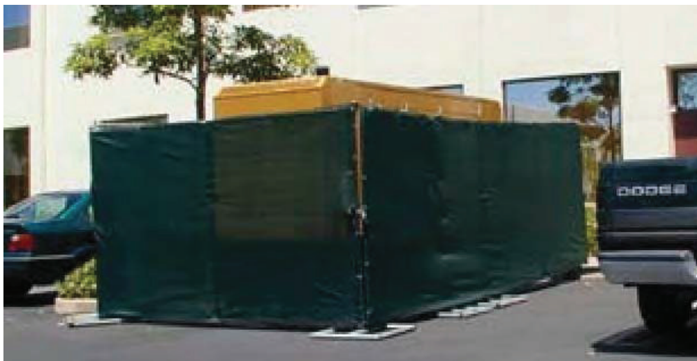
Figure 5-26 Example of Inappropriate Ground Mounted Equipment Screening
