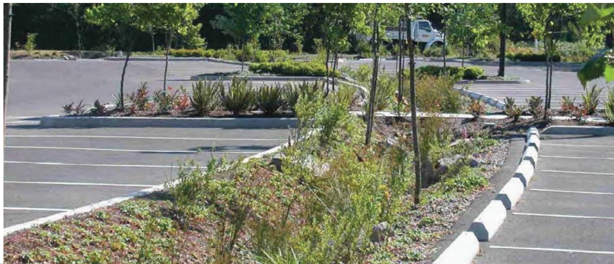
Figure 5-7 Example of Biodetention Facility
