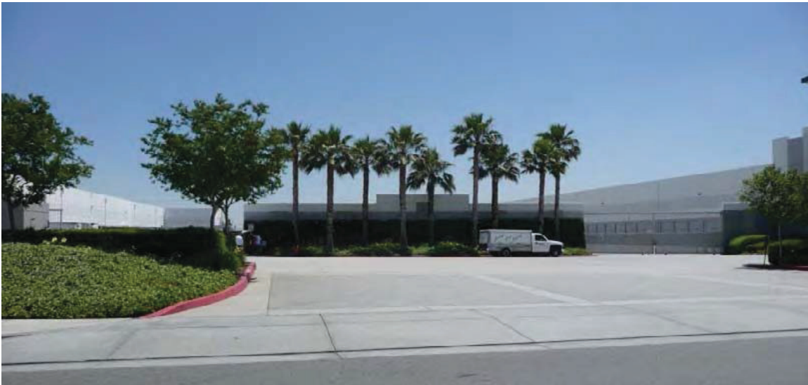
Figure 5-25 Example of Appropriate Ground Mounted Equipment Screening
