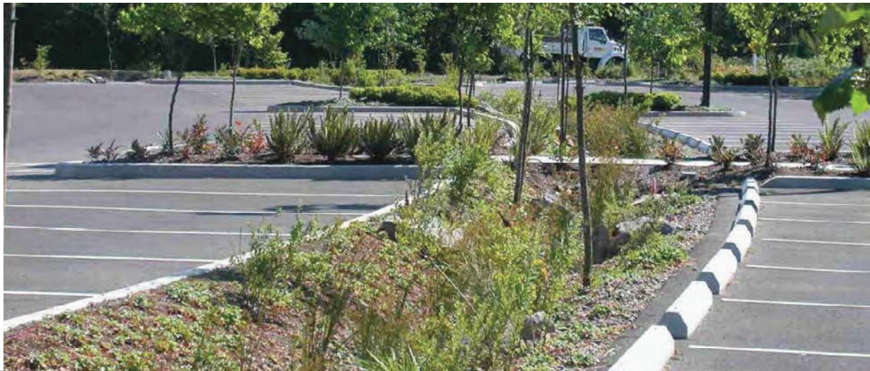
Figure 5-7 Example of Biodetention Facility
