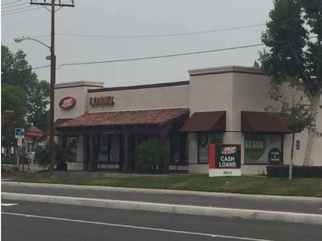
View of the adjacent property to the northwest
