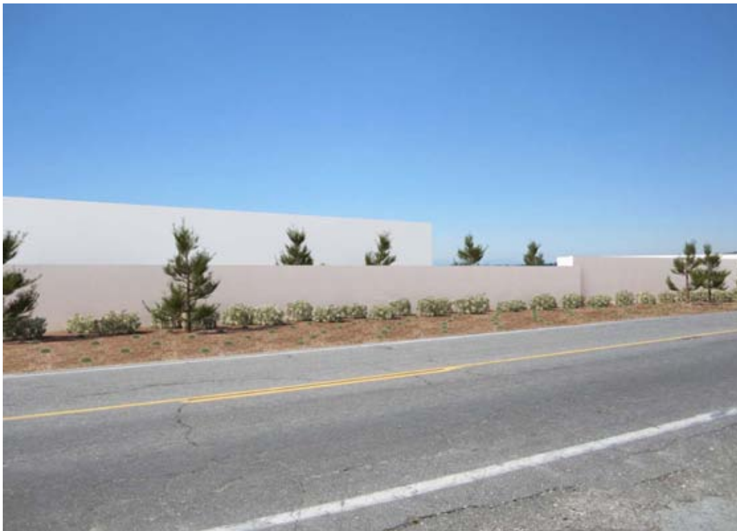
Gilman Springs Rd. View 5 at Installation
