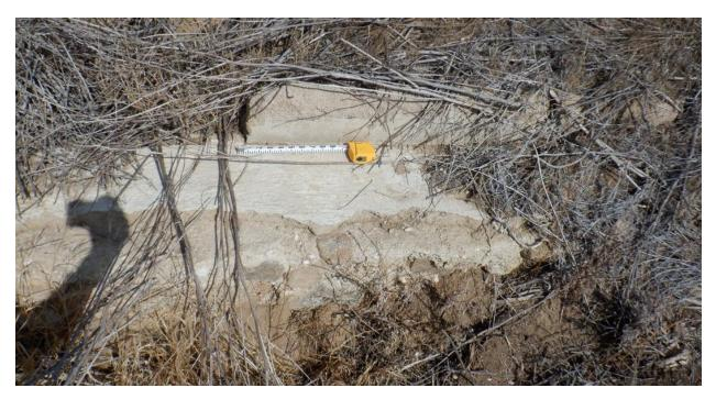
Photo 3. Mid-section of concrete irrigation channel and mortared rock wall. (Michael Baker International 10/13/2022)
