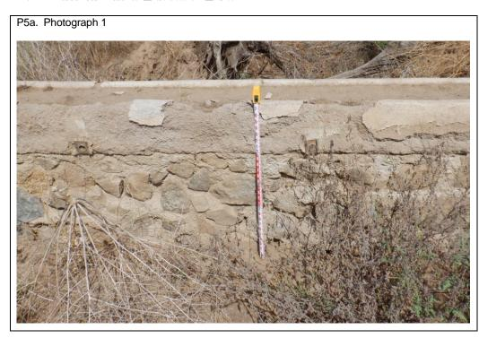
**P5b. Description of Photo:** Photo 1: Segment of elevated concrete irrigation channel and mortared rock wall. View north. 10/13/2022
