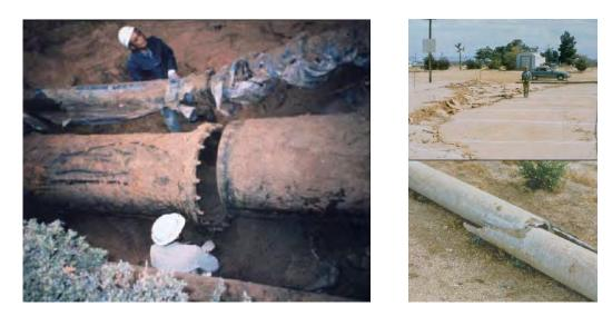
The photograph on the left shows a pipe joint pullout due to liquefaction from 1995 in Kobe, Japan. (photo courtesy of D. Ballantyne, *Understanding the Seismic Vulnerability of Water Systems*, Regional Water Providers Consortium Board, October 2013)
