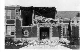
The 1933 M6.7 Long Beach earthquake took place on March 10 at 5:54 P.M. Damage to buildings was widespread and between 115 and 120 people died. The earthquake highlighted the need for earthquakeresistant design for structures in California.
