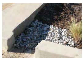
Figure 2: Curb Cut located in a Bioretention Facility
