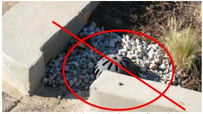
Figure 6: Incorrect Placement of an Overflow Inlet.
