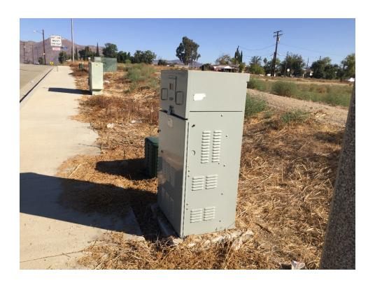
Photo 11: Two electrical control panels adjacent to the two pad-mounted transformers along the western boundary of the Property.
