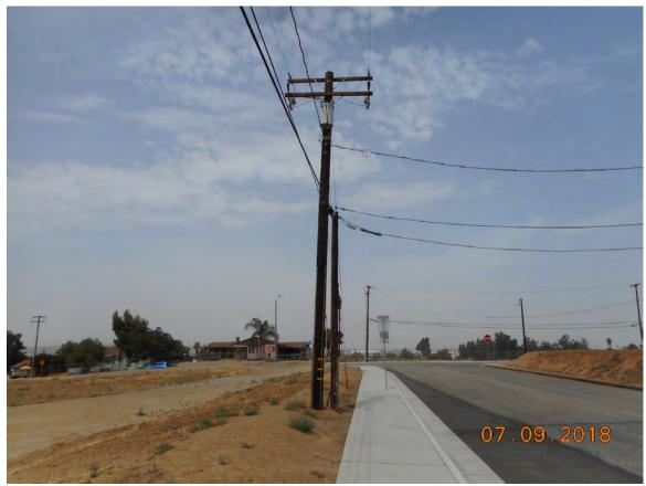
PHOTO 9 - VIEW FACING WEST TOWARDS THE NORTHWEST SUBJECT SITE CORNER, STANDING ALONG THE SOUTH SIDE OF SHERMAN AVENUE. NO LEAKAGE WAS OBSERVED AT THE POLE-MOUNTED ELECTRICAL TRANSFORMER SHOWN IN THE FOREGROUND.
