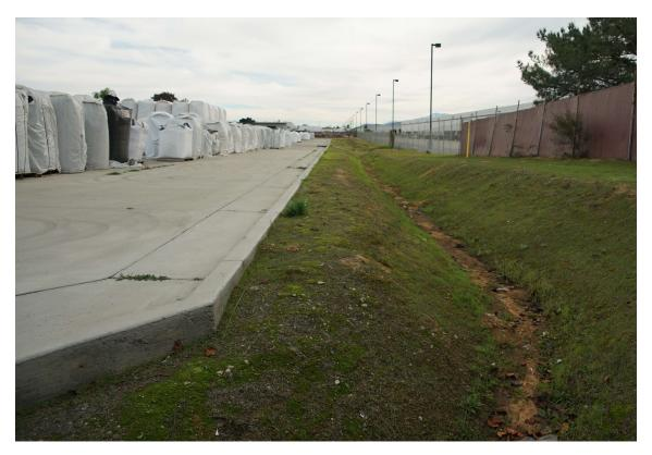
**Photograph 1** Southern Property Line - Looking East. Developed Area - linear maintained detention basin
