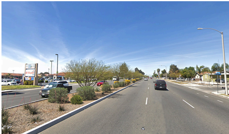
Alessandro Boulevard is six-lane road with a center median and a bike lane in some portions
