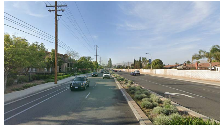
Frederick Street near Towngate Boulevard. The street has four lanes, a center median, Class II bike lanes and six-foot wide sidewalks. Perimeter walls and fences line the street along residential developments.
