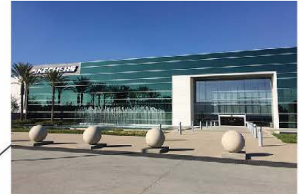
Skechers Distribution Center
