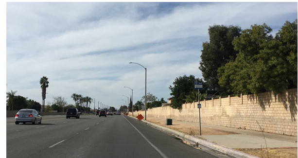
Perimeter wall along the street
